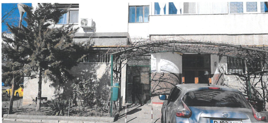
F5. Usa acces principal in bloc
